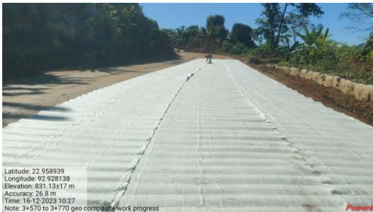
Geo Composite Work Progress
